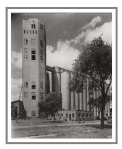
The Midway elevator (later Bunge) was among the early structures, at 12<sup>th</sup> Ave. SE and the Great Northern tracks. It was a wood structure that was expanded several times, most significantly in 1936-1937, when the tower and new row of elevators were built of reinforced concrete. The Bunge Midway elevator continued in operation until 2003.
